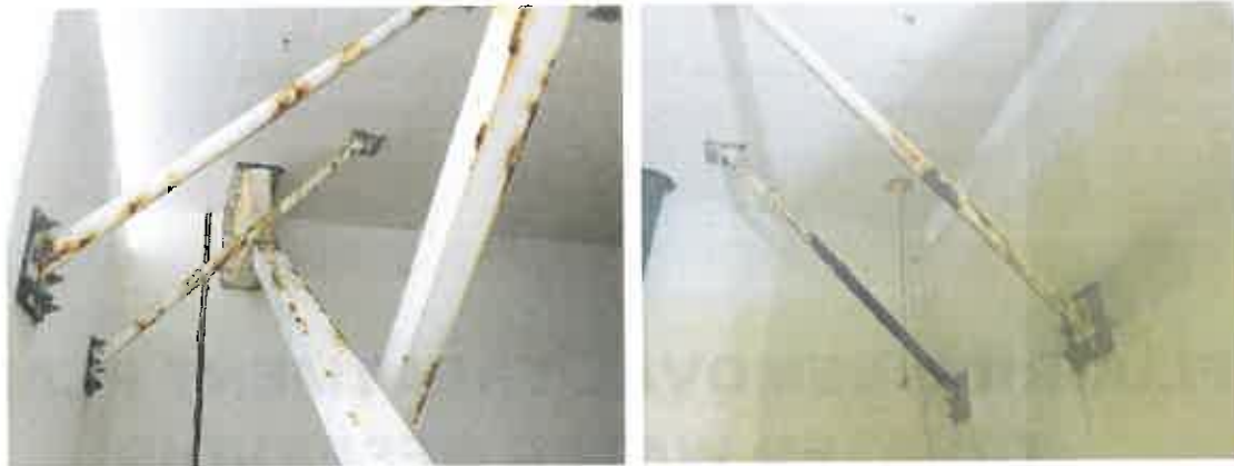
Figure 1: Internal Steel Braces
